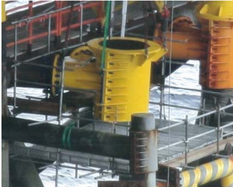
Completion of top riser clamp (+5 m) installation at CKR platform
