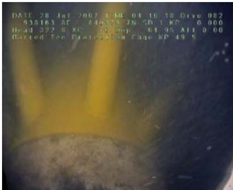
Completion of Barred Tee protection cage installation at KP49.5
